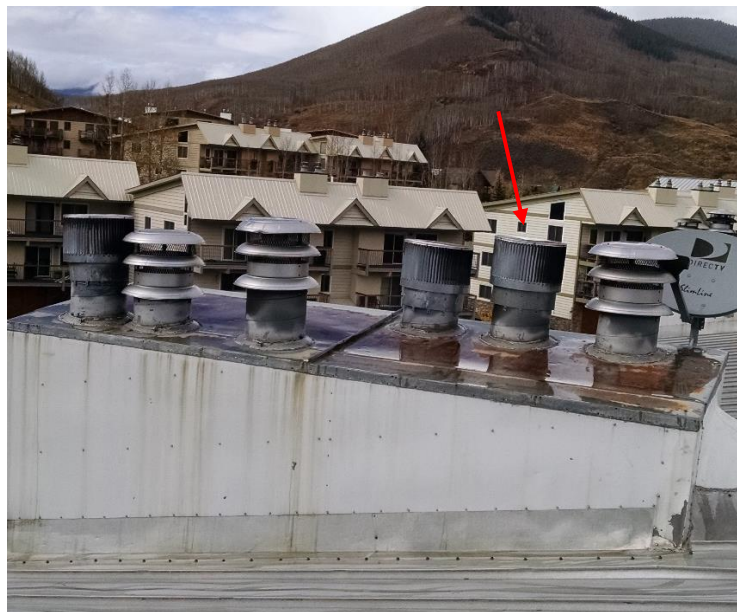
Manufactured Chimney System
