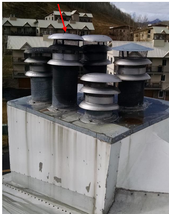
Manufactured Chimney System
