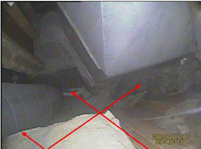
Insulation touching chimney & fireplace, a 2" airspace is required No firestop provided where chimney passes through floor/ceiling
