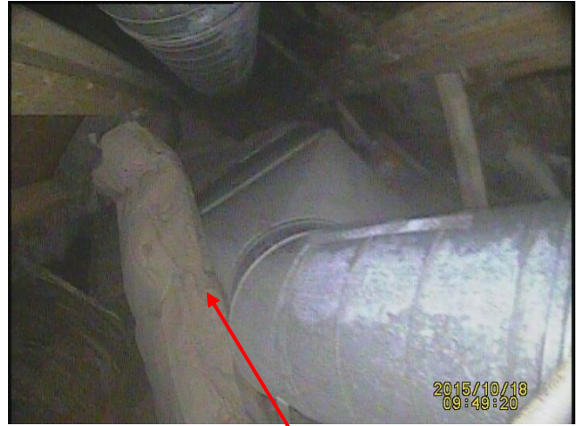
Insulation has fallen on top of a fireplace. This is a serious fire hazard
