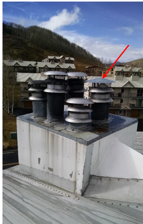
Manufactured Chimney System
