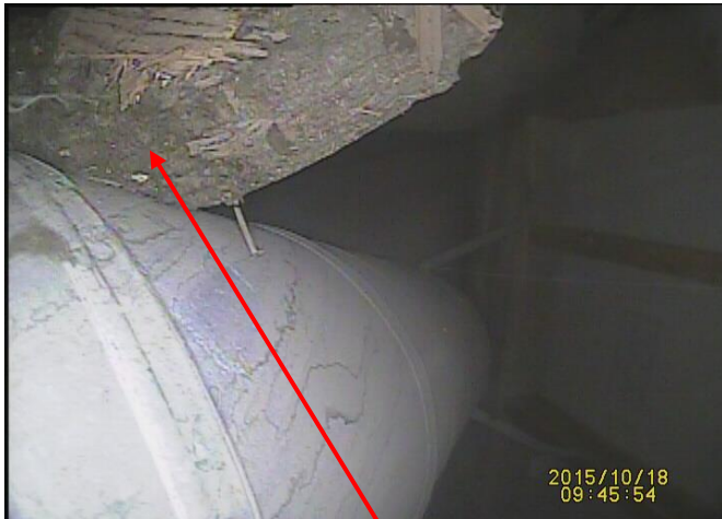
Combustible building material in direct contact with the chimney. This is a serious fire hazard
