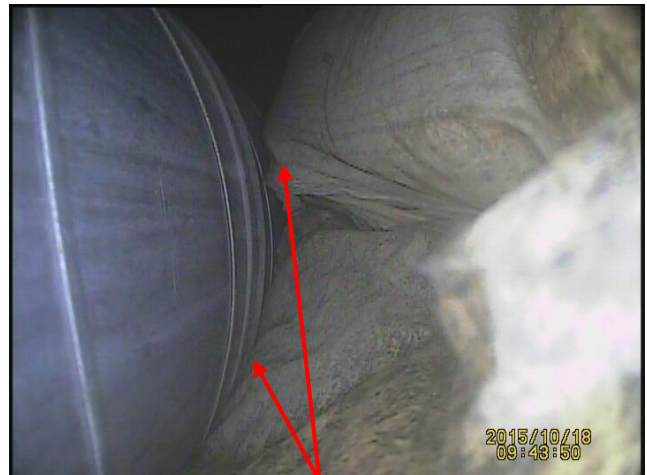
Combustible insulation in direct contact with the chimney. This is a serious fire hazard
