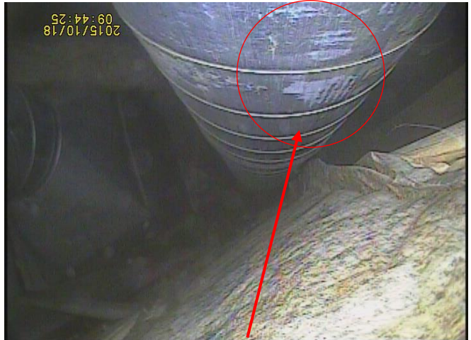
Signs of moisture damage on the outer wall of the chimney
